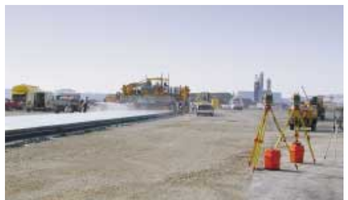
Machine operator Beat Furrer is relieved of control chores by the Leica Geosystems machine guidance system (white box) fitted in the driver's cab – not unlike the aircraft guidance systems which pilots now take for granted. Now he can concentrate wholly on the production process: “Our taxiways are absolutely perfect!”.
