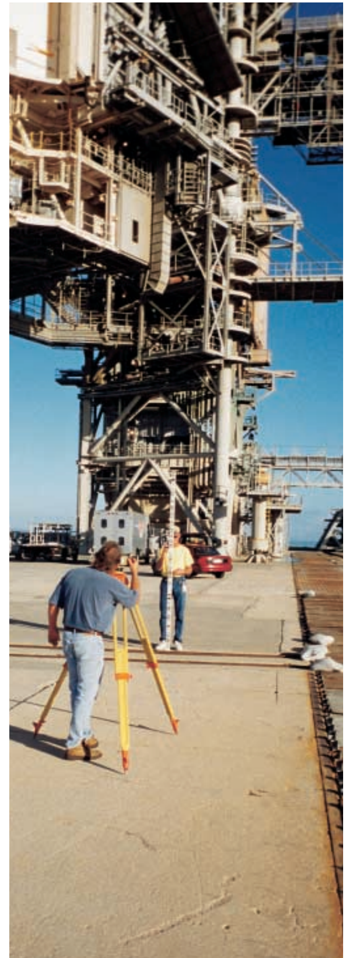
Left: Donald Lanthorne, perched at a dizzying height to check the elevation of the gaseous oxygen vent using a Leica NA 3003 digital level, and (right) measuring the RSS rails with Kevin Beuer.
