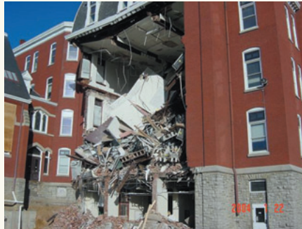
The geometry of collapsed buildings can be captured in detail with a high-definition survey.
