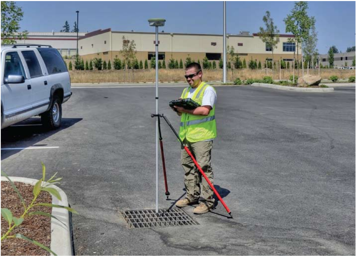
The CH2M HILL crew also used MobileMatriX in conjunction with the Leica GPS 1200 RTK unit.
