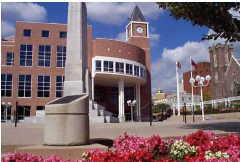
▲ On the outskirts of Toronto, Brampton is among the largest and fastest-growing urban centers in Canada. Its Engineering & Construction Division's Surveys & Mapping Section supports $80 million annually in major capital reconstruction.
